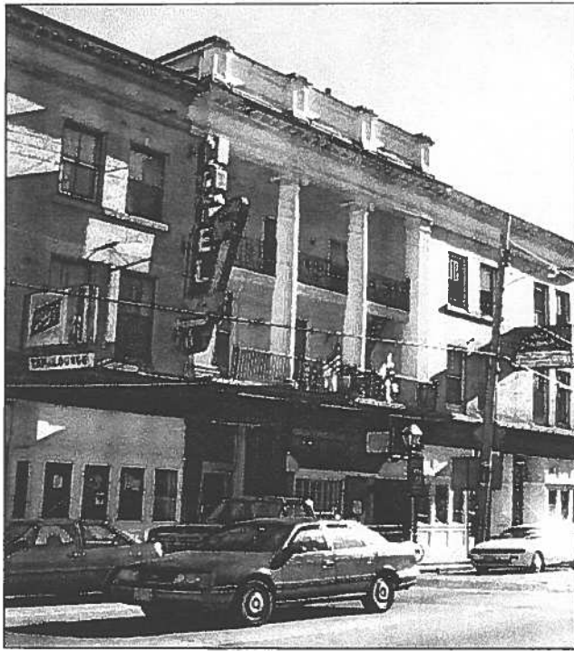
The historic Greenwich Hotel, pictured above, is currently under restoration, and upon completion, will be a major asset for Main Street. Streetscape improvements will enhance this asset.
